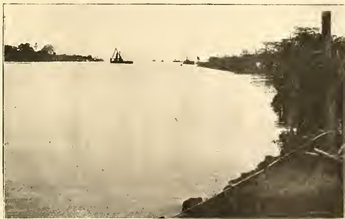
PART OF THE COMPLETED CANAL
